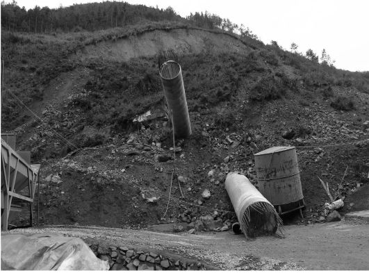
图 1 滑坡推倒公路桥基柱 Fig. 1 Landslide Pushes Down Pile Foundation of Expressway
