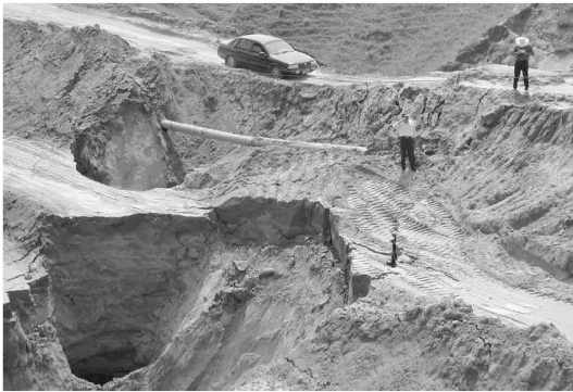
图 3 黄土洞穴引起的路面塌陷(环县) Fig. 3 Pavement Collapse Created by Loess Caves(Huan Xian County)
