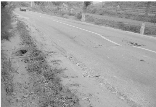
图 2 暗穴引起的路面凹陷(吴旗—志丹) Fig. 2 Pothole Created by Loess Hidden Hole(Wuqi—Zhidan Highway)
